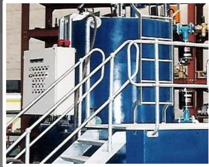
Control panel with PLC and integral cable racking
